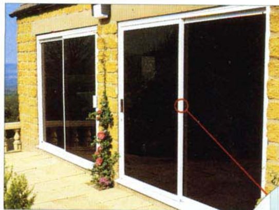
Ⓖ When closed, the sliding panel (1) interlocks with the fixed panel to prevent them being levered apart.
